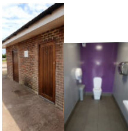
Refurbished toilets at Market Yard car park
