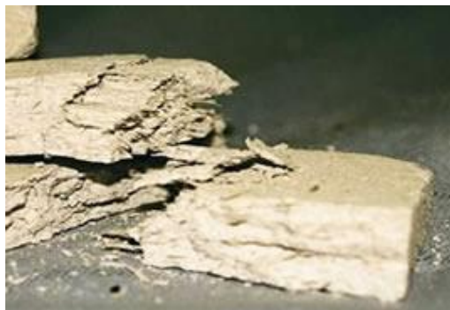
Pieces of Asbestos Insulating Board (AIB)
