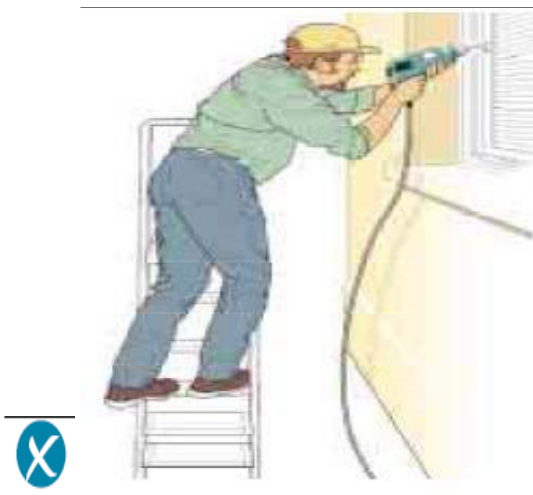
Incorrect – steps side on to work activity
