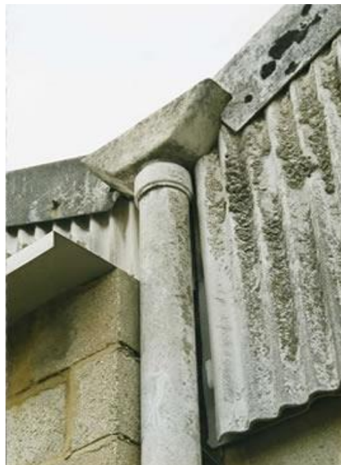
Asbestos cement downpipe, hopper and profile sheet
